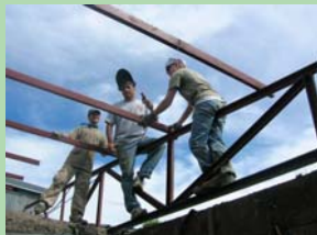
And a New Roof!
