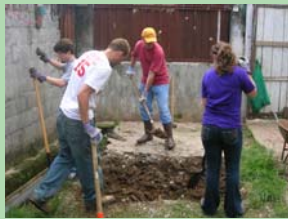
A New Septic Tank
